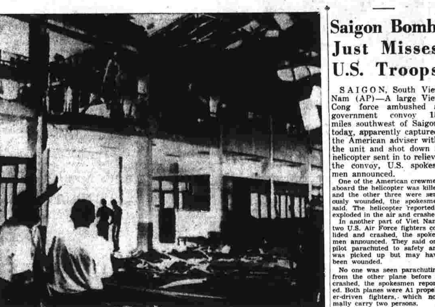
Debris hangs from the roof and litter the floor of the Saigon airport damaged yesterday by a terrorist's bomb. Every window in the structure was blown out by the explosion. (AP Photofax.)
